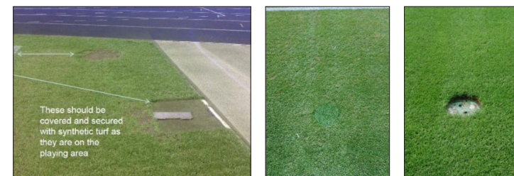
Fig. 28. Access and service boxes within the safety zone around the field of play
