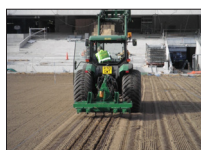
Fig. 7. Installing undersoil heating pipes through the profile
