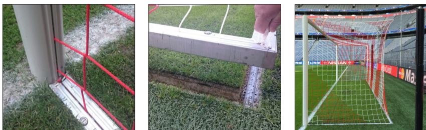
Fig. 24. Goal frames recessed into the ground. If screws or any other elements used to support the goal structures are deemed a potential hazard, additional protection such as tape or padding must be used (Fig. 25)
