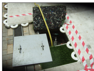
Fig. 91. Quick coupler valve access points, allowing ground staff to irrigate areas that need it (turf exposed to sun or wind).
