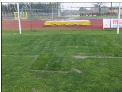
Fig 37. Poor surface levels in a re-turfed goalmouth.
