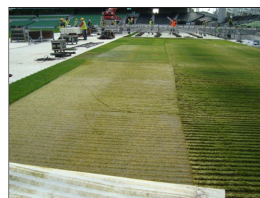
Fig. 88. Aluminium trackway panels used to allow heavy vehicle access onto the pitch, with and without removing the turf first. On the left, significant damage was done to cool-season turf after 11 days of panelling; on the right, the turf was removed prior to installation and the panelling laid on a geotextile surface.
