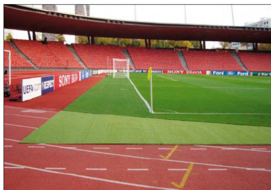
Fig. 27. Extension of turf perimeter around the field of play using high-quality artificial turf
