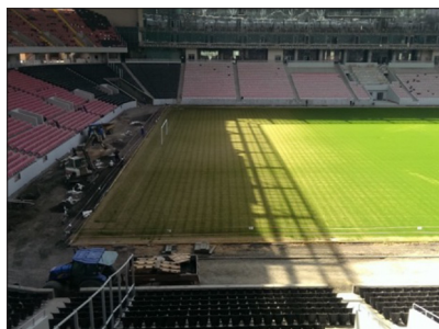
Fig 49. Effect of shade on turf establishment – artificial lighting rigs will be essential in winter to maintain growth.
