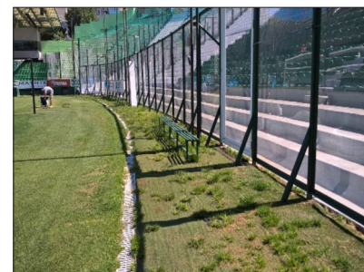
Fig 37. Lack of weed control on artificial turf perimeter leading to poor aesthetic appearance.
