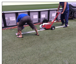
Fig. 18. Wheel-to-wheel line marking following a string line (left) and marking out dashed lines (right)
