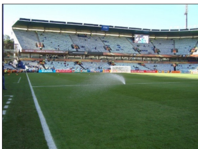
Fig 37. Irrigation system with low sprinkler pressure – leads to poor irrigation coverage.
