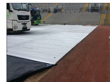
Fig. 88. Aluminium trackway panels used to allow heavy vehicle access onto the pitch, with and without removing the turf first. On the left, significant damage was done to cool-season turf after 11 days of panelling; on the right, the turf was removed prior to installation and the panelling laid on a geotextile surface.
