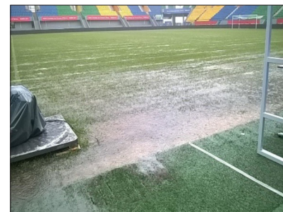
Fig 37. Heavy rainfall on a pitch with poor surface drainage – such conditions can lead to matches being abandoned.
