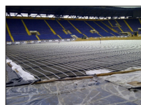
Fig. 6. Racks used over the gravel drainage layer to support undersoil heating pipes prior to root-zone placement
